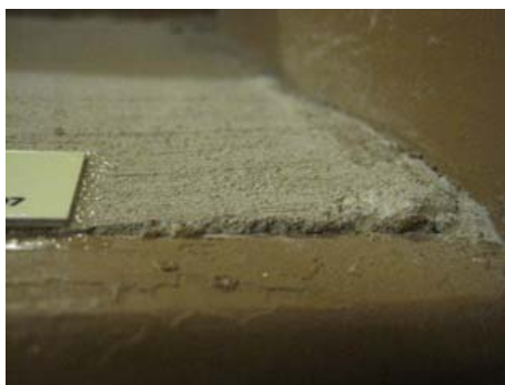
Rising Concrete right before side wall
