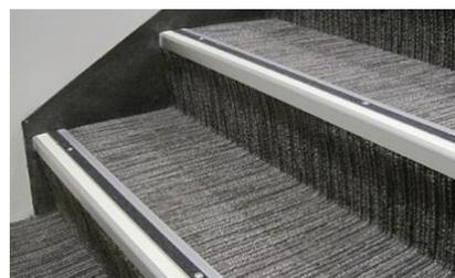
Drill through the black anti-slip tape channel to firmly attach the 90° angled Aluminum Nosing to the carpeted Step Edge. Use a black Sharpie pen to blacken the silver-colored screw heads to blend them in with the black Anti-Slip Tape.
