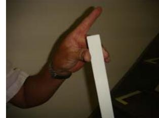
8. **Position alu marker 1/2 inch away from leading edge of step. Do NOT install right on the front edge of a step or landing. Do NOT round or curve the alu strips. An adhesive strengthener, such as Loctite Heavy-Duty Construction Adhesive or LiquidNail<sup>®</sup> may be used for extra adhesion. This is especially important on diamond plate surfaces or steps with channels or grooves.**
