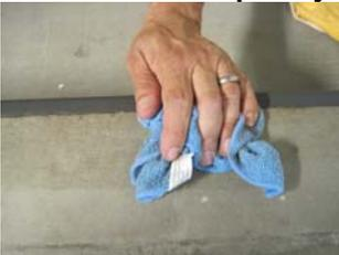
4. Once the water-cleaned surface has dried, wipe installation surface with **70% Isopropyl alcohol**, using a different micro-fiber cloth. Let the Isopropyl alcohol evaporate completely. Prior to material installation the surface must be dry, dust-free and clean.
